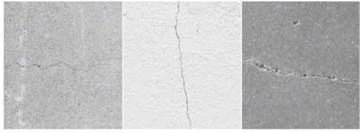
Diamond Design Precast reinforces all our products with steel reinforcement for certifiable structural integrity. However, even the best concrete installations will sometimes see hairline cracking in finished precast concrete products. It's
